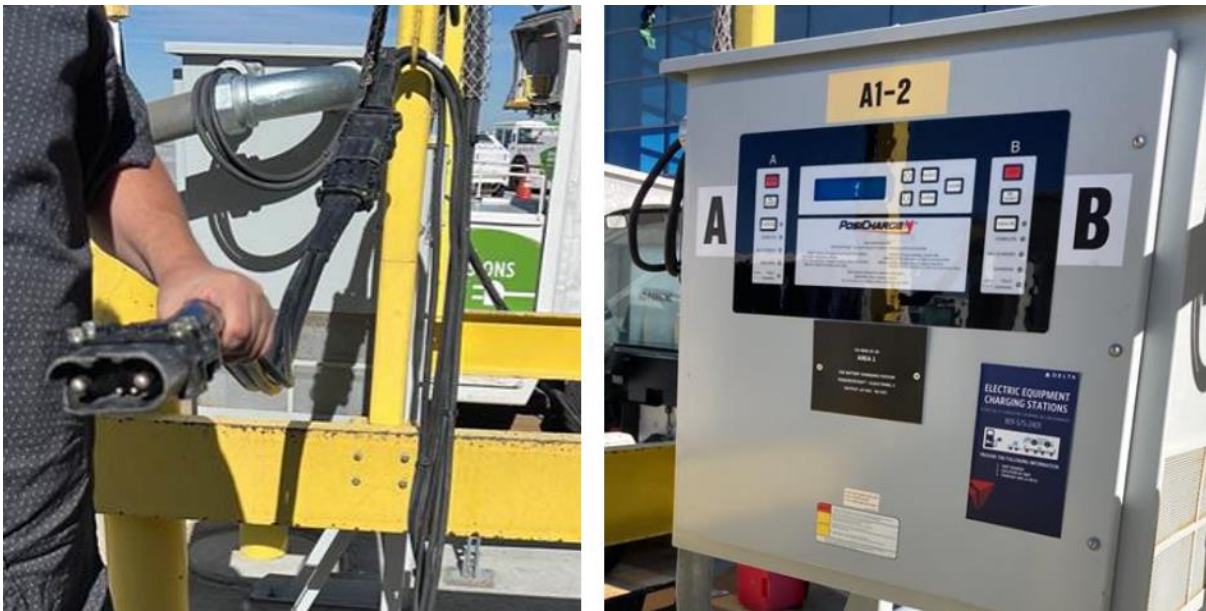
Figure 4: Posicharge mvs800 charger for SLC airport tugs. [23]
