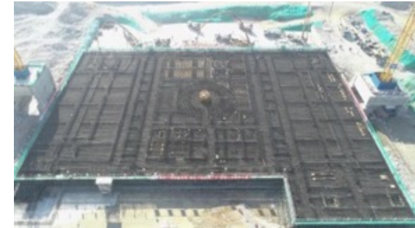
Construction site of CFR-600 – source WNN
