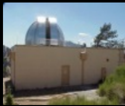
Ground Laser Transmitter (GLT) Table Mountain, CA 1m-OCTL Telescope (5 kW)
